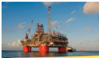
Thunder Horse: BP’s largest production and drilling platform in the Gulf.
